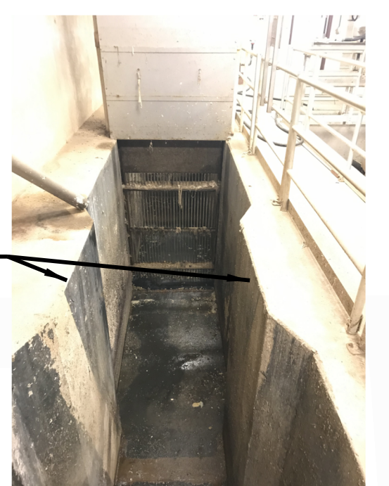
PHOTO OF LOWER LEVEL COARSE SCREEN CHANNEL BELOW ALTERNATE SCREEN LOCATION
