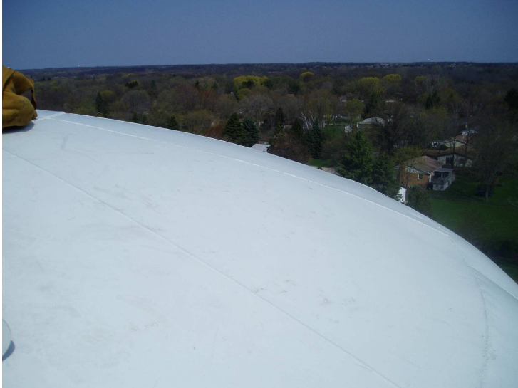
27) View of the roof coating.
