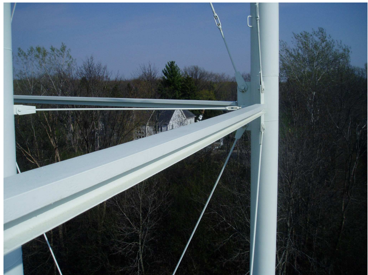
17) Looking at the struts and sway rod connection to the leg.
