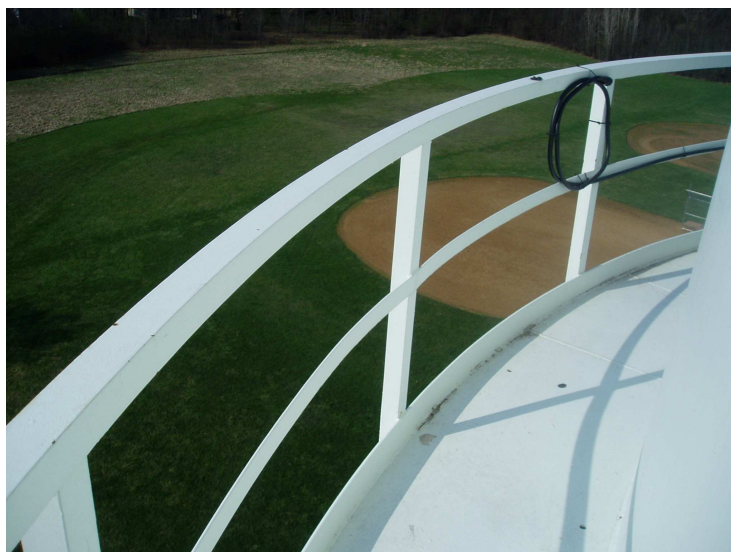
21)View of the balcony handrail.
