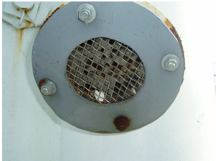
14) Looking at the screen on the overflow.
