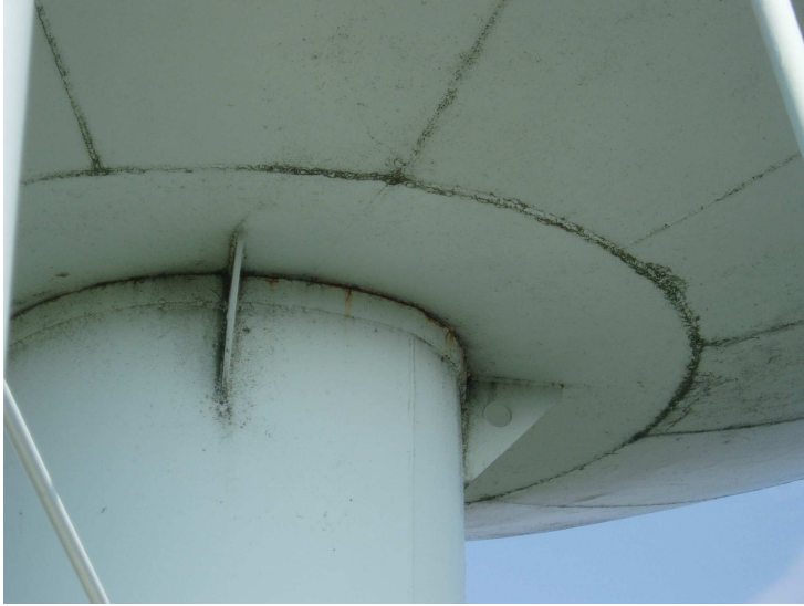
19)Riser connection to the bowl is in good condition.
