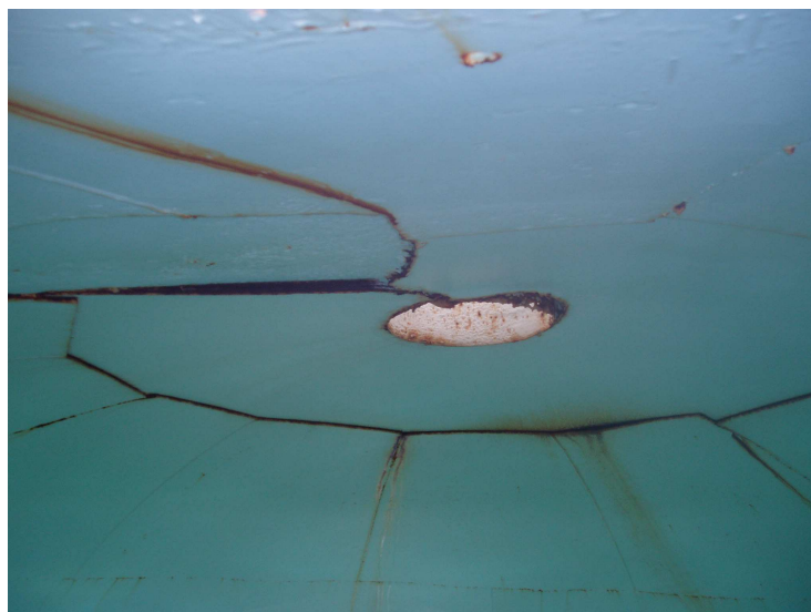
32) The wet interior roof coating is in fair condition.
