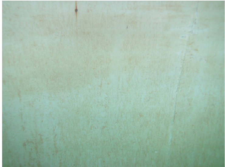
37) The coating on the roof knuckle is in good condition.
