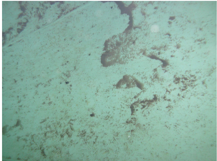
40) The coating on the lower sidewalls is in good condition.
