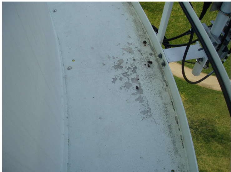
20)Spot coating delamination on the balcony floor.
