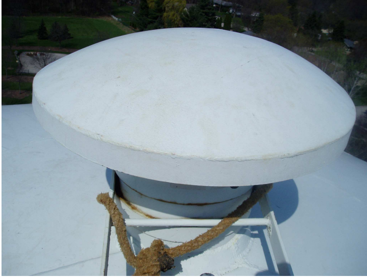
30) The roof vent is in good condition.
